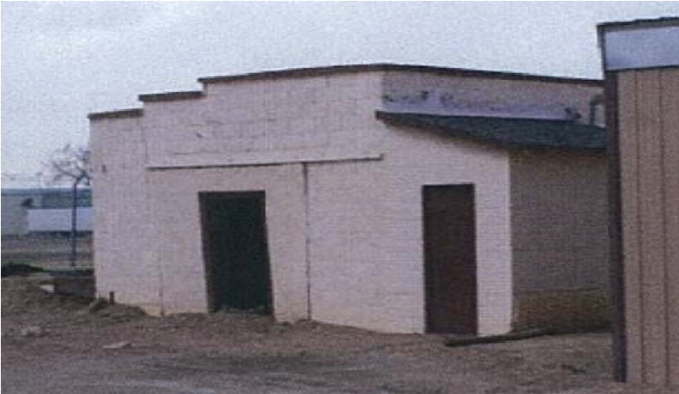
Building 2 Concrete block – isn't really usable.
