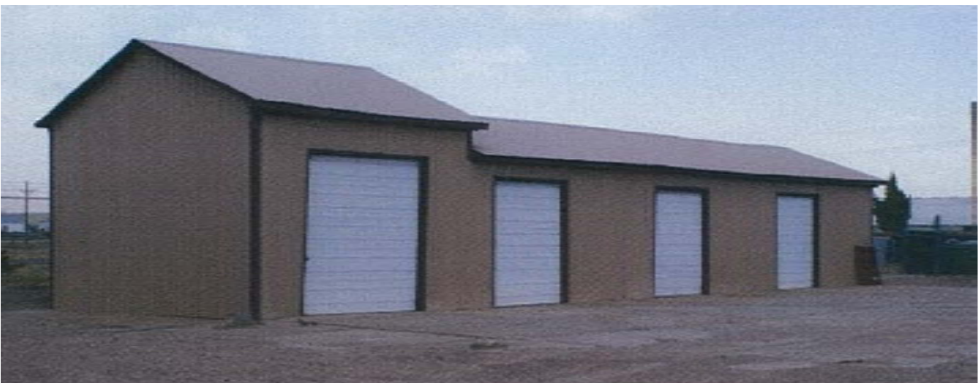
Warehouse (building 4) 1,00 sq. ft., frame, metal siding, 4 overhead doors, cold storage.
