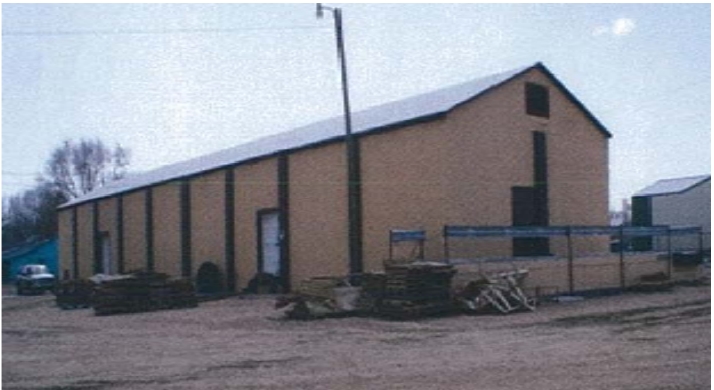
Warehouse (building 1) 3,280 sq.ft., Concrete block, 2 overhead doors, separate office/secure storage area. All cold storage, no heat.
