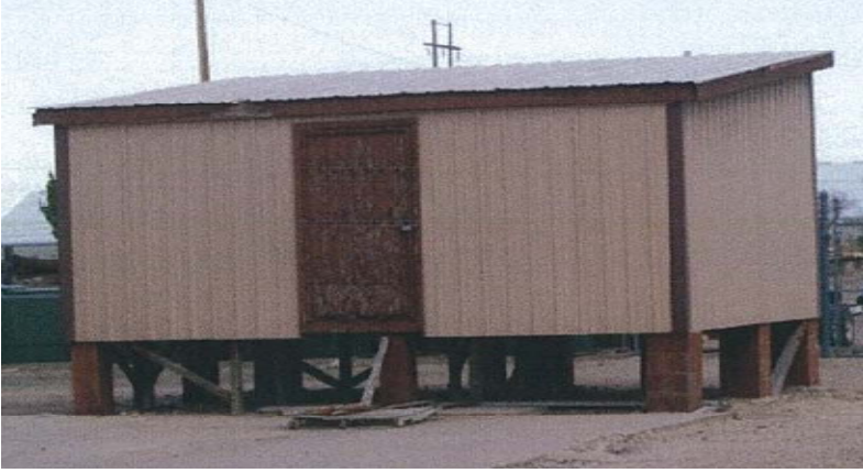
Warehouse (building 5) 315 sq.ft., frame, metal siding, on risers, 1 hinged door, cold storage.
