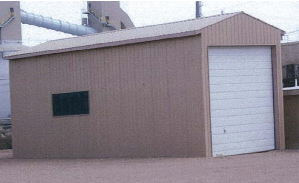
Garage next to office (building 6) 1,104 sq. ft., frame, metal siding, 3 overhead doors, cold storage.
