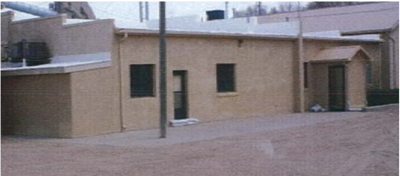
Office (building 7) 5,869 sq. ft., concrete block, stucco, GFA/CA, multiple office stations, lots of built-in desks and storage, restroom facilities, kitchen/break room, reception area, storage closets, 3 outside access doors.
